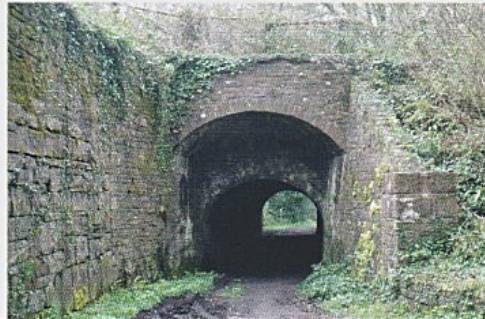
Clydach Railroad tunnel (2019) Twnnel Rheilffordd Clydach (2019)
