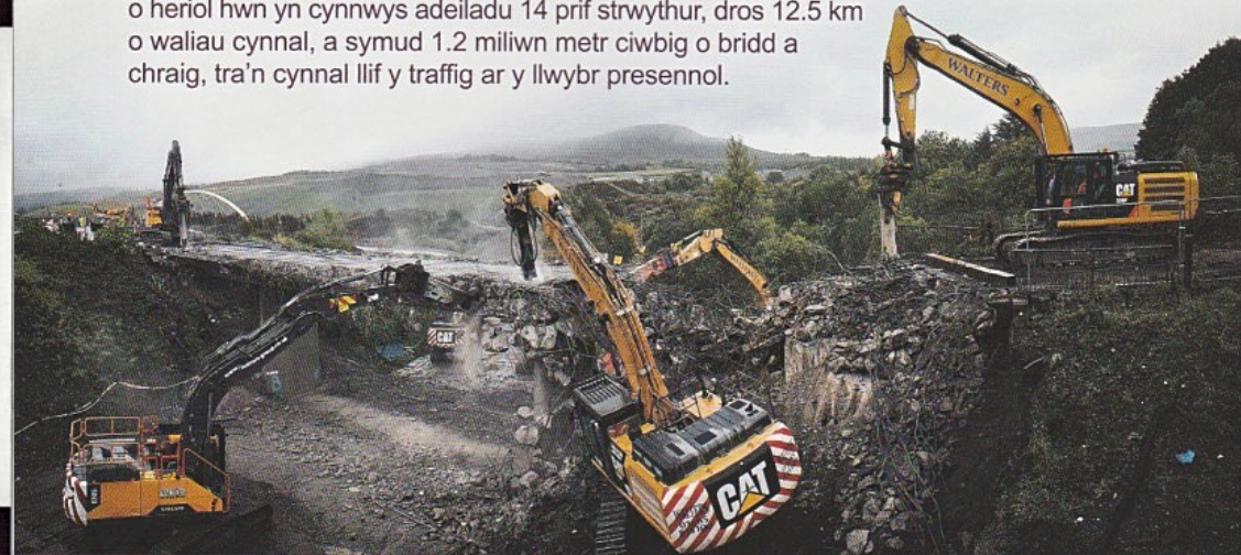
Demolition of Intermediate Road bridge (2018)
