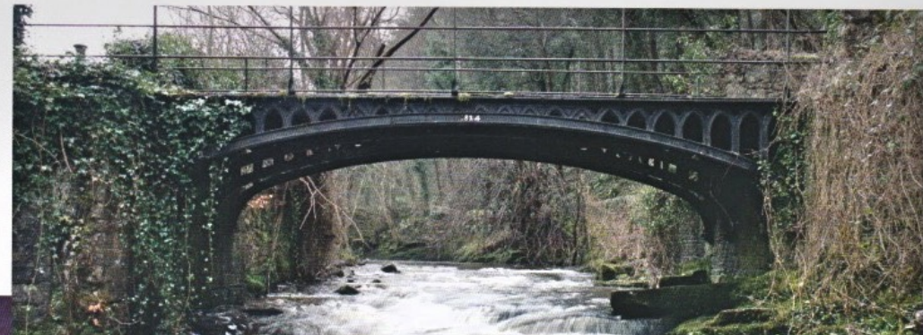
1824 tramroad bridge over the River Clydach (2019)
